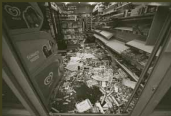
Damaged shop, Croydon
