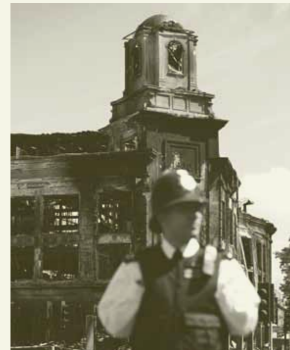
The burnt out remains of a building, Tottenham, London
